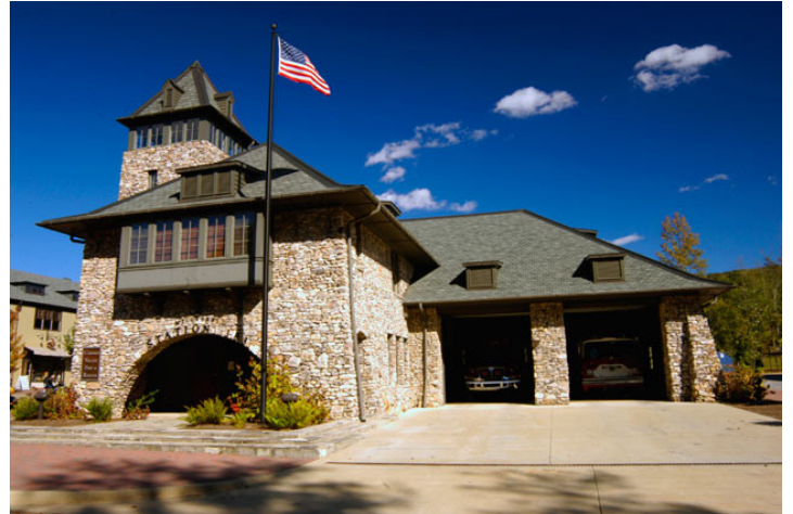
Mr. Laurel fire station
