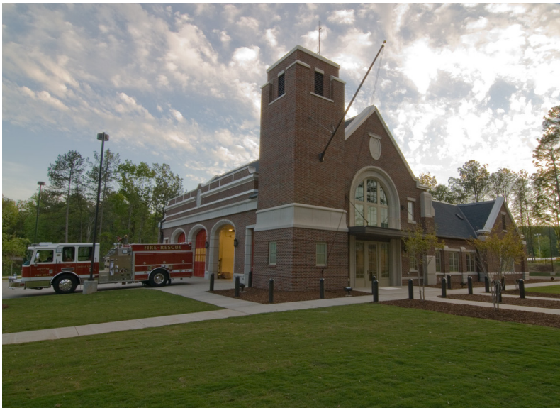
The Preserve fire station in Hoover.
