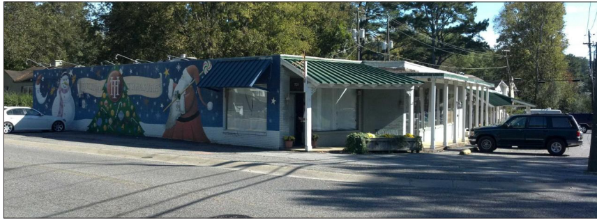
Existing conditions at retail building across from Patriot Park
