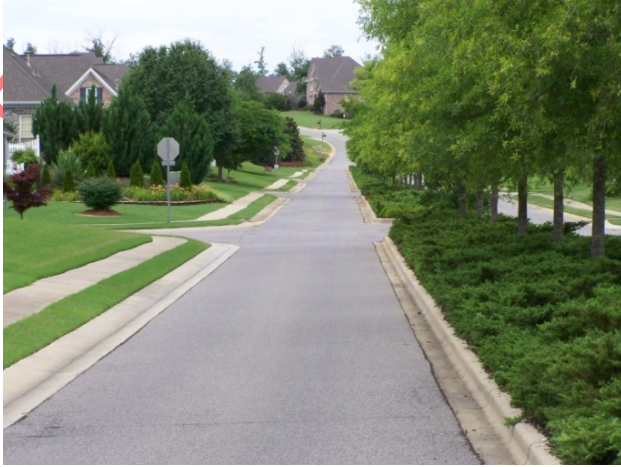
Sidewalks, median and street trees - Clay, AL
